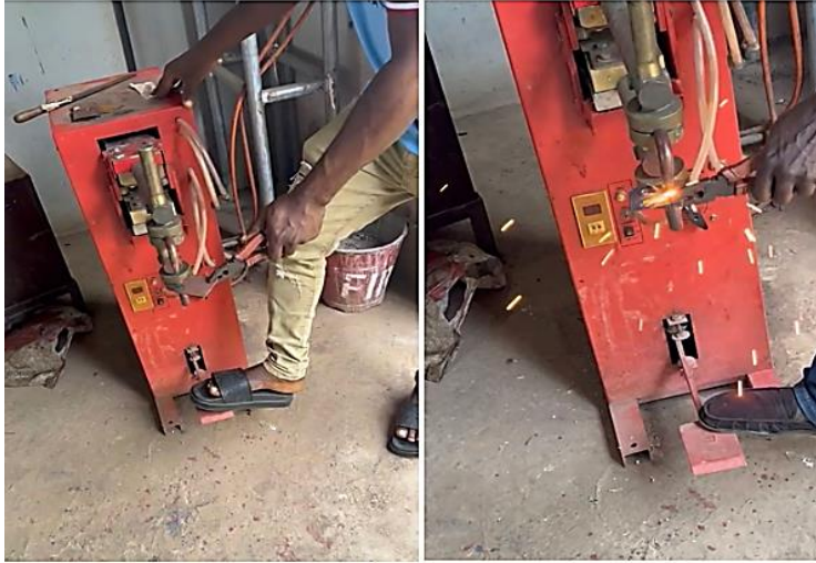
Fig. 1: Welding of 1 pass
